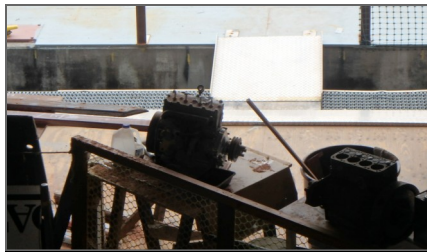
Air Start Engines for Compressors
