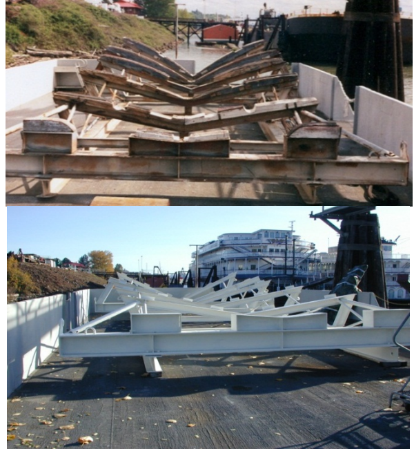
PT Boat Cradle on Barge, Before and After
