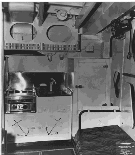
PT631 Builders photo shows galley stove
