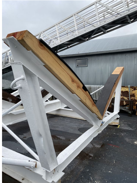
Photos above of cradle show exposed steel where bunks will be replaced (left), and new replacement bunk (right).
